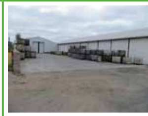
Fish Oil now contained and stored properly
