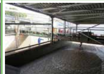
Upgraded Fish Pits with fencing and extended roofing at Westpoint Processors
